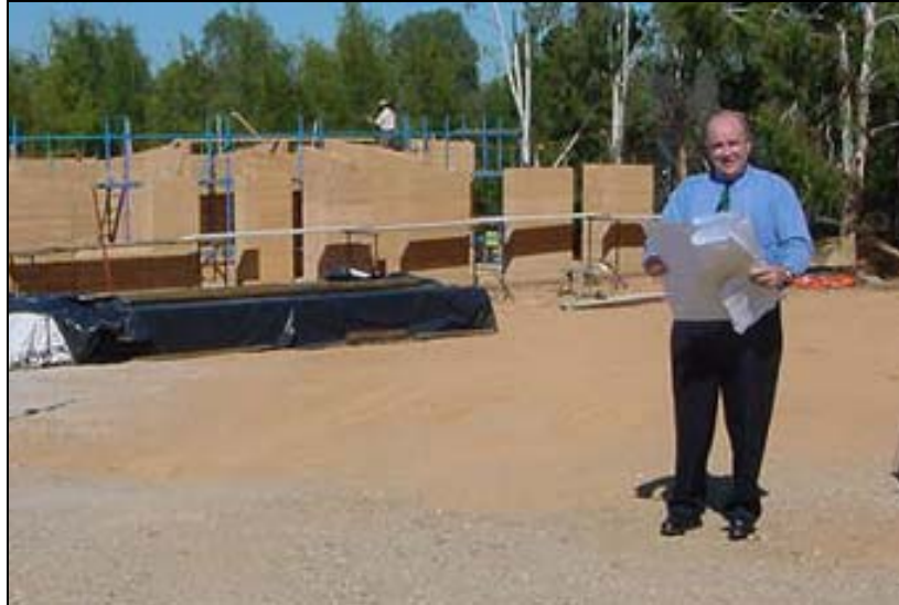
Construction of Residential Cottages
