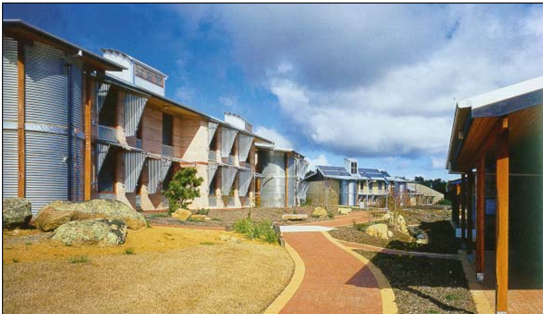
SEIS office building with Lecture Theatre Complex in background
